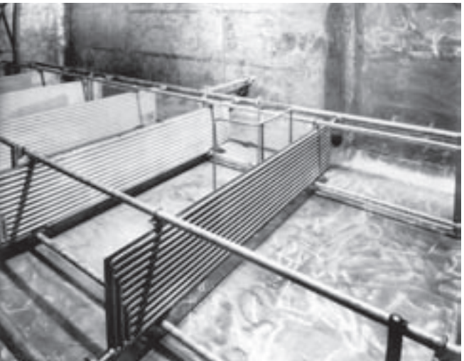
Fig. 65-3 The stainless steel PLATECOIL shown here are in a large compartment of a food products tanker. They are used for heating or for cooling depending on the product being transported.
