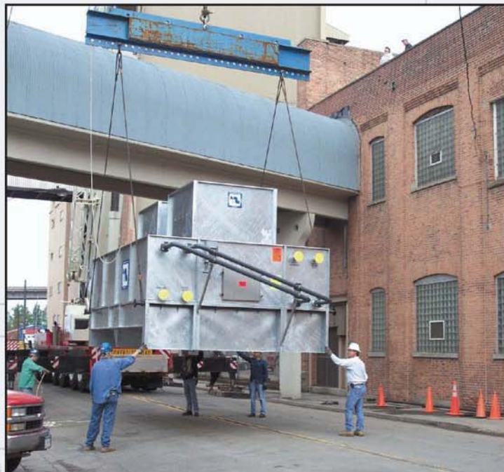
Modular equipment installation
