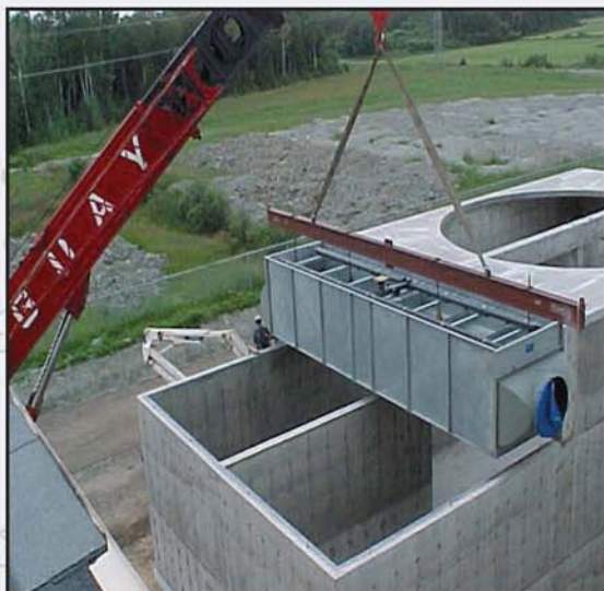
Field erected cells
