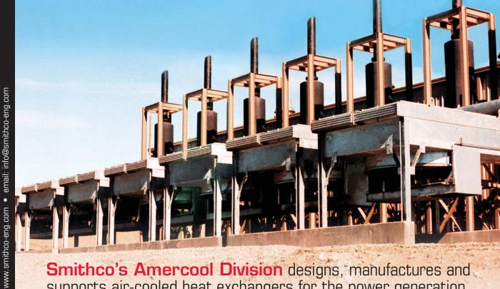
Smithco's Amercool Division designs, manufactures and supports air-cooled heat exchangers for the power generation industry. Applications include radiators, generator sets, landfill gas cooling as well as others.
