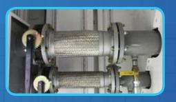
Piping coolant lines are protected with braided stainless steel, flex-connectors and butterfly shutoff valves.
