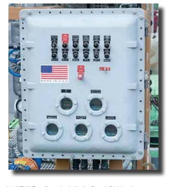
A typical NEMA Type 4 panel for areas temporarily exposed to combustible gases. Panel is equipped for Type Z pressurization and also purges the small panel on the left.
