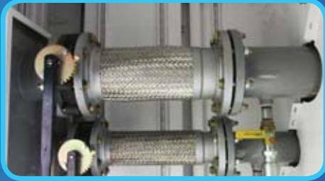
Piping coolant lines are protected with braided stainless steel, flex-connectors and butterfly shutoff valves.
