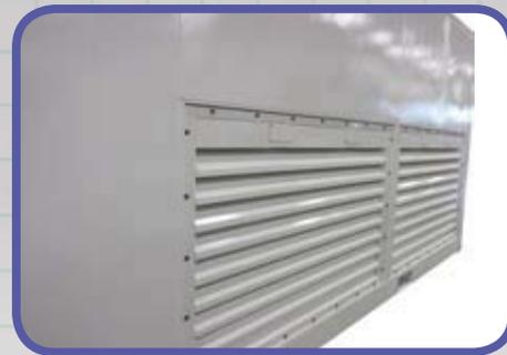
Louvered panels are easily removed, providing access to both motors and fans.
