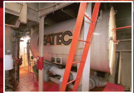
Heatec 10-million Btu/hour heater installed below-deck on an asphalt barge. The barge holds 44,000 barrels of liquid asphalt and regularly travels the Great Lakes.
