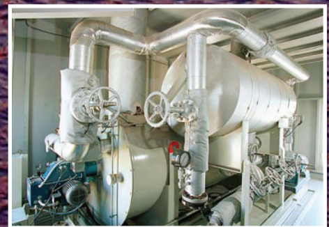
Heatec 2-million Btu/hour heater installed above-deck on a phosphate barge.
