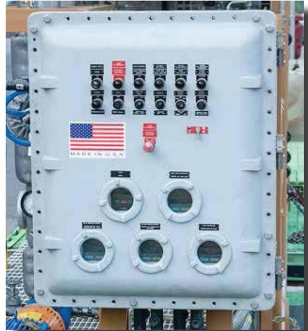
A typical NEMA Type 4 panel for areas temporarily exposed to combustible gases. Panel is equipped for Type Z pressurization and also purges the small panel on the left.
