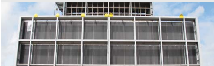
Gas Turbine Inlet Air Cooling
