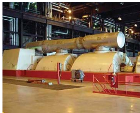
Multiple pressure balanced expansion joints
