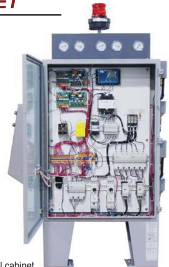
Titan electrical cabinet
