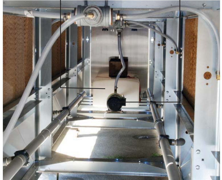
Internal view of Hydra II Fluid Cooler
