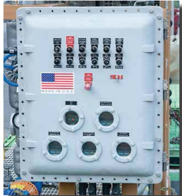
A typical NEMA Type 7 panel suitable for Class I, Division 1 areas. These panels can also be used for Class I, Division 2 areas to eliminate the need for purging.
