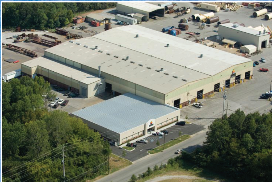
Heatec facility in Chattanooga, Tennessee
